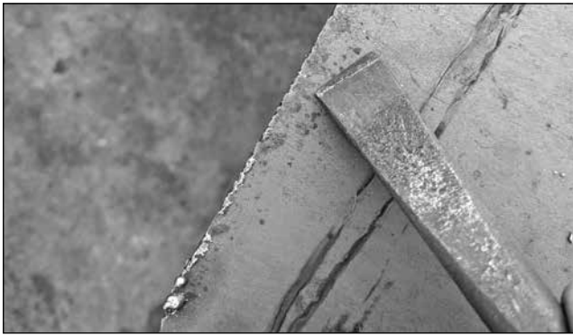
I chisel away most of the slag at the cut
