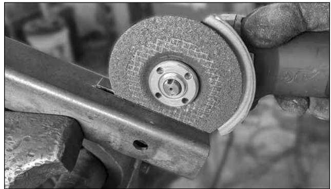
Use a "Zip" disc or other suitable media to cut the slots into the side of the outer legs
