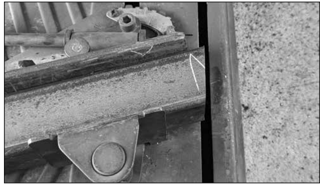
Cut the end of all the legs to 15°. The cuts are parallel not opposite. Weld seam up or down
